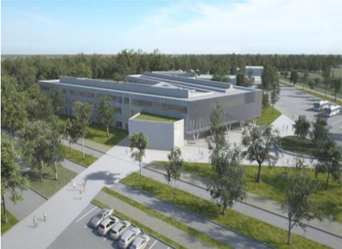
Photo: Nort-sur-Erdre high school project - Establishment selected for the ADEME «E + C» call for proposals, aims to obtain certification of the NF mark «Tertiaires buildings – Démarche HQE® (high environmental quality)in the ADEME's "E+C" call for projects, and aims to obtain NF "Tertiary Buildings –HEQ" (high environmental quality) certification
